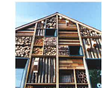
Mellor Primary School by Sarah Wigglesworth Architects
