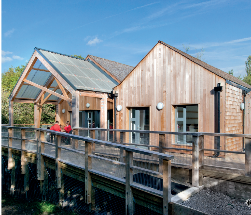
The building's construction makes use of natural and reclaimed materials, including straw bale insulation, timber off-cuts and even car tyres
